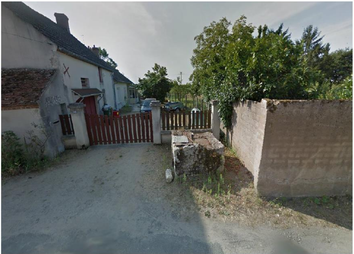
Puits (Source : Google street view, 2012)
